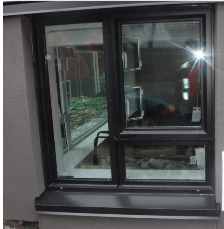
Example of triple glazed vinyl framed window with casement operable vent
